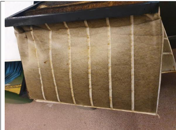
Filter change/duct inspection 03.03.2020
